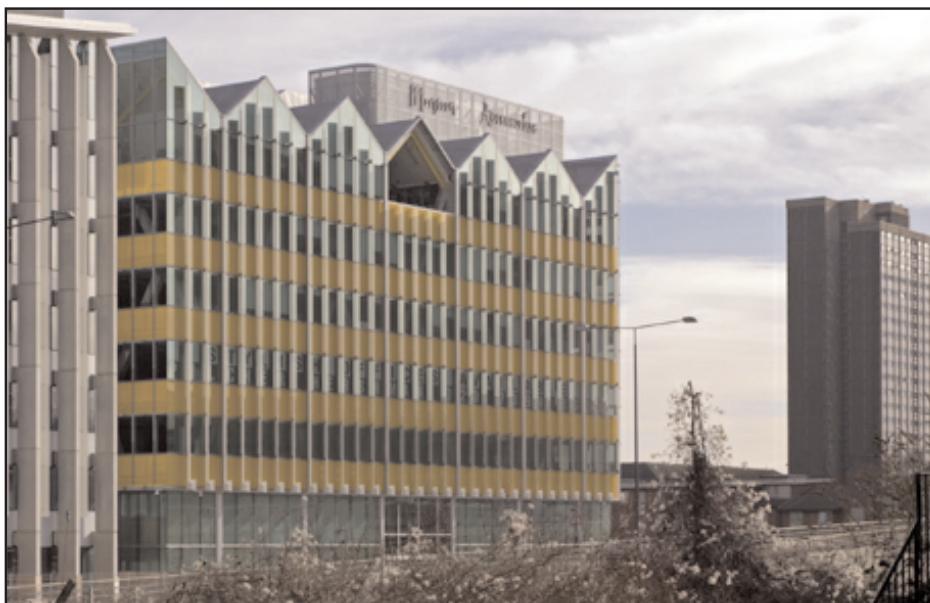
Is this what creatives want? A new breed of good-looking, low-spec space. The Yellow Building, Notting Dale, W11, has been described as a "white collar factory" targeted at creative users. It was commissioned by fashion retailer Monsoon and designed by AHMM. Agents are Pilcher Hershman.
